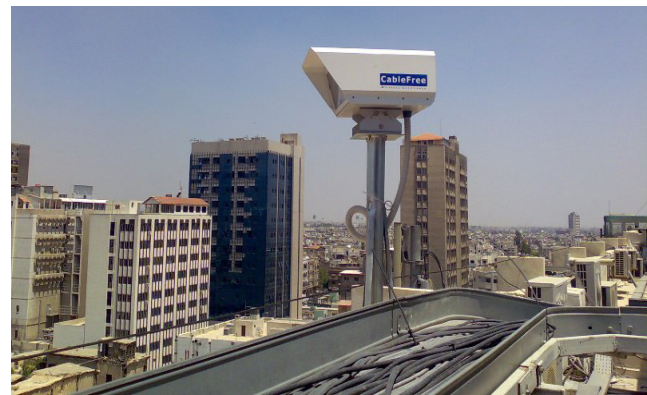
Figure 4: FSO installed in the Middle East
