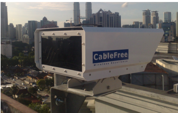
Figure 3: FSO installed in Malaysia
