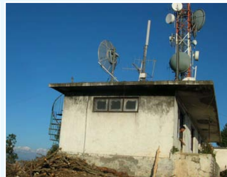
Nagarkot Repeater Station
